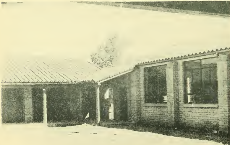
In The Patio With Detailed View Of Cinder-Block Masonry And Gray-Back Tile Roof.
